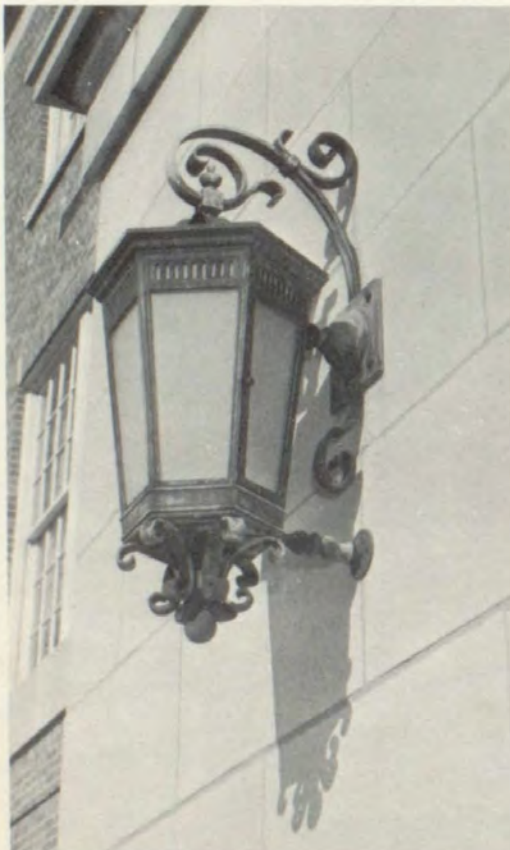
Lighting the entrance
